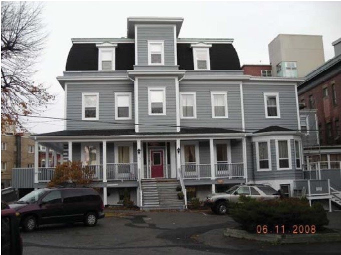
First Steps Housing Photo Courtesy of Housing Alternatives
